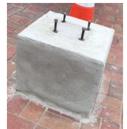
Smithville Sculpture on Main Concrete
